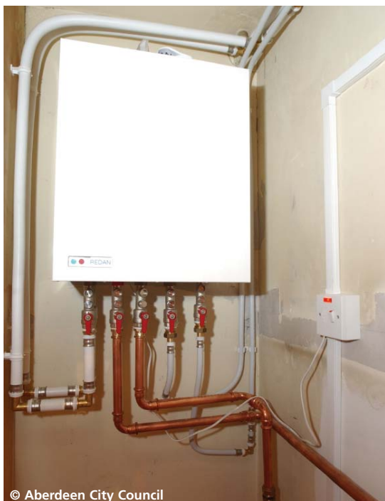
Figure 3: A heat exchanger inside one of the flats
